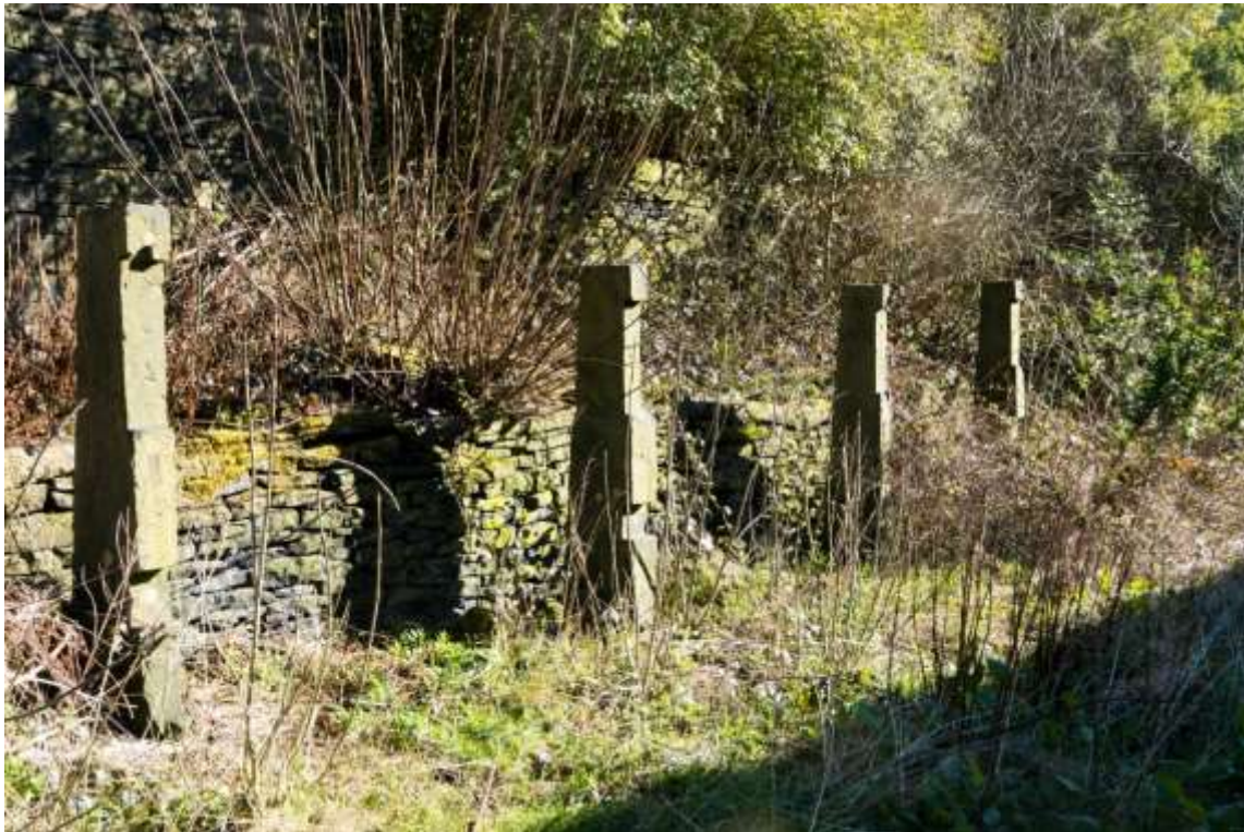
Figure 8. Stone tenter posts at Marsden, West Yorkshire, probably early 19 th century. They are sited in an urban setting outside a large mill. Note the slots for adjustable tenterhook beams.
