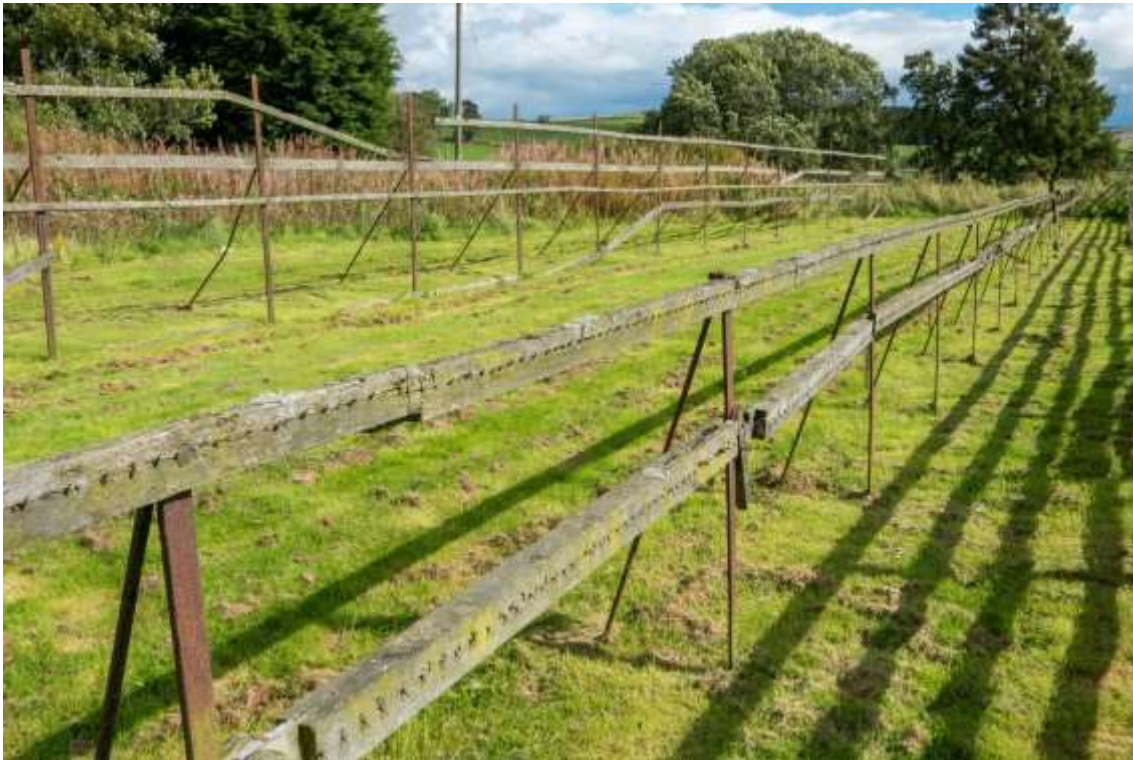
Figure 1. Tenters at Otterburn Mill showing the two seams for different cloth widths.
