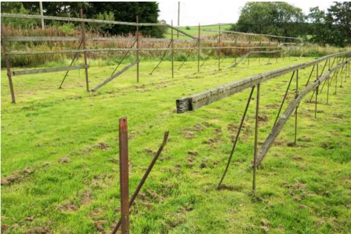
Figure 3. Damage and missing sections to parts of the two seams in 2017. There has been further damage due to recent flooding.
